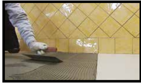
Fig.28 - This method refers only to adhesives that bear the indication "single-layer" by the manufacturer. Spread adhesive on the complete surface of the support. Follow the instructions of the manufacturer of the adhesive as regards type of spatula and spreading methods.
