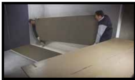
Fig.31 - To handle tiles, raise them to their upright position, whilst grasping them from the top edge. They can then be moved with the help of a second person.
