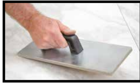
Fig.30 - After laying the tile, make sure it is firmly bound to the underlying surface to prevent gaps and air bubbles forming. For this purpose you must use a tile beater with a rubber bottom (for example Raimondi "142G").
