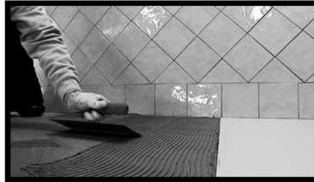
Fig.62 - Floor installation
