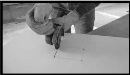
**Fig.19** - To obtain internal and L-shaped corners, round off the vertex of the corner using bits with a radius of at least 5 mm that reduce the risk of breakage. Then cut with diamond discs, taking care to stop moving the cutting tool forward when you reach the hole previously drilled. To drill and cut using diamond discs, follow the instructions provided above.
