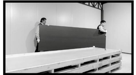
**Fig.3** - When the slab is upright, hold it from its top edge and shift it keeping it straight and upright. This operation should be performed with the aid of a second person.
